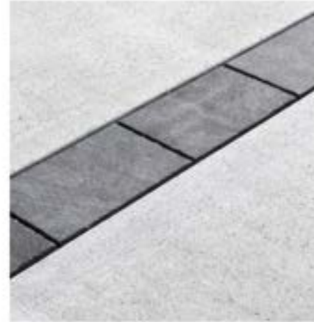
DRIVEWAY MATERIAL CONCRETE WITH PAVER BOARDER
